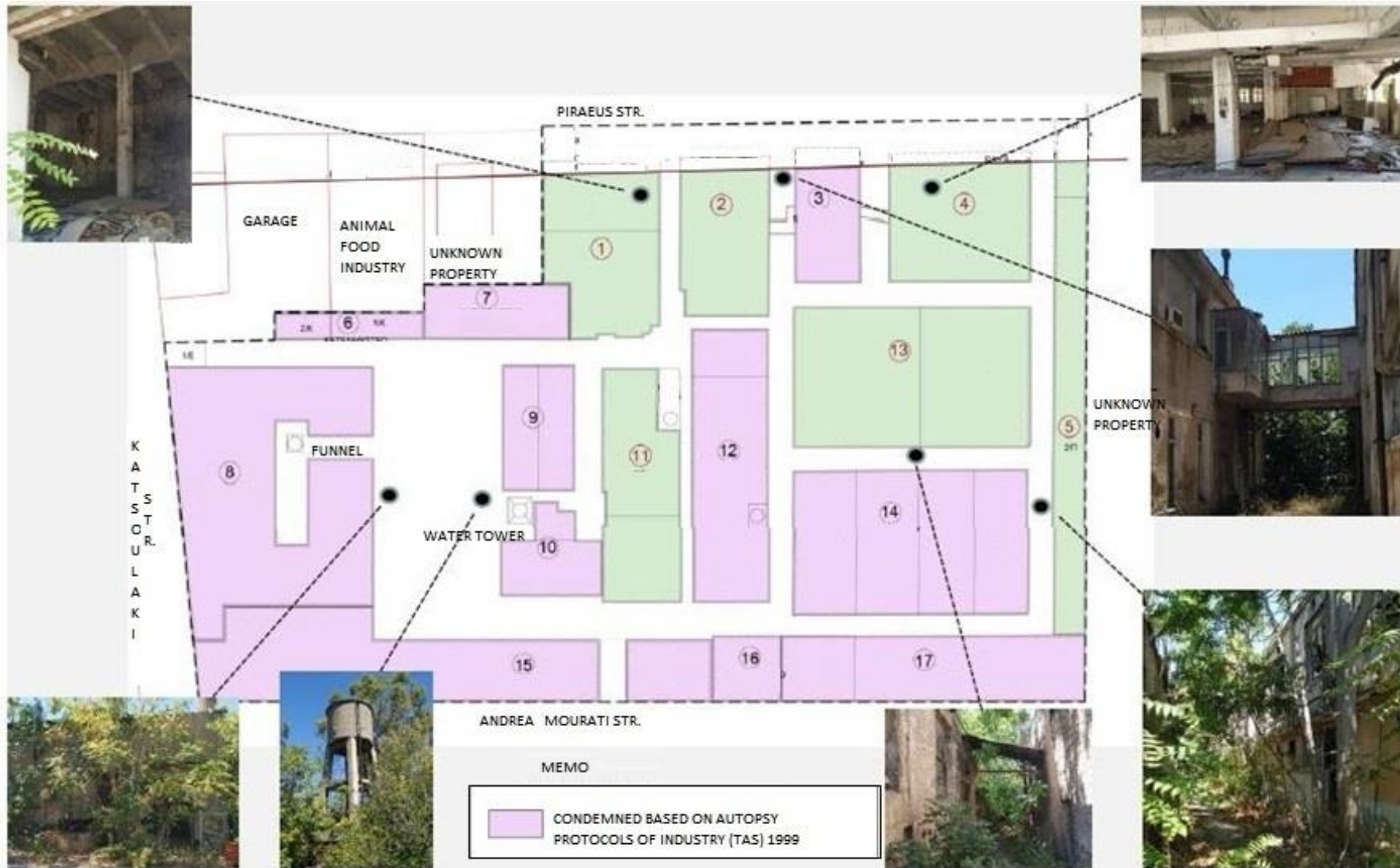
Image 3: Current condition of the Property
